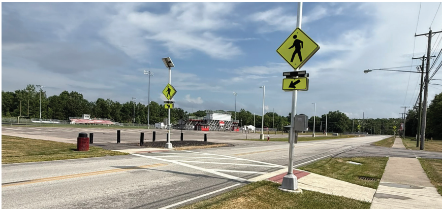
FIGURE 3 Existing crosswalk on Harris Road
