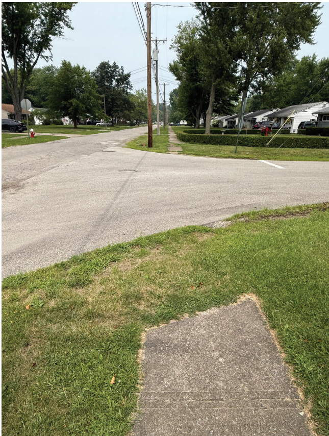
FIGURE 13 Many streets have incomplete or narrow sidewalks that do not connect well to intersections with crosswalks. This example is of the intersection of Forestlawn Avenue and East Drive.
