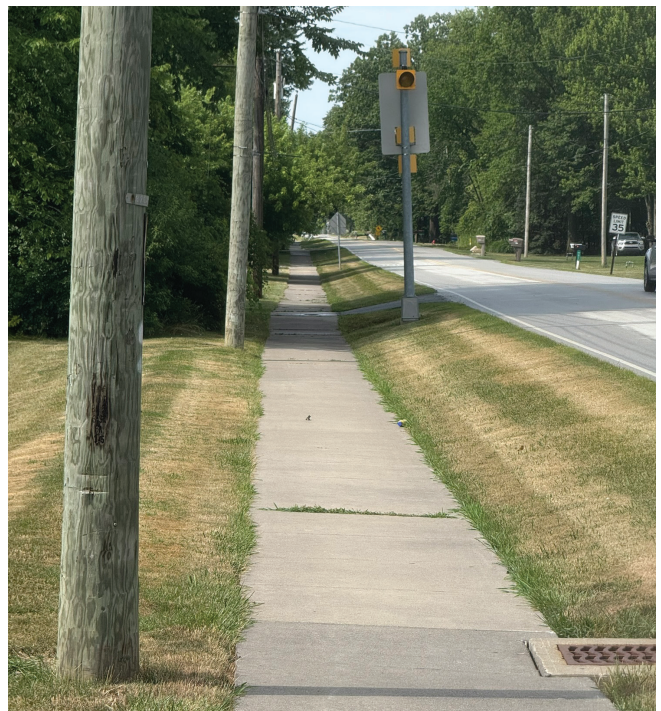
FIGURE 15 Newer sidewalks, like the ones on Harris Road, are separated from the curb by a buffer of grass to increase comfort.
