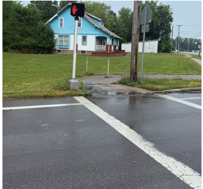
FIGURE 17 Many major street crossings have a signal to stop traffic and a pedestrian countdown timer, like this intersection of Harris Road and Colorado Avenue. Still, many crossings feel uncomfortable, either because of factors like poor sidewalk connectivity on either end, water pooling on curb ramp, and standard placement markings (instead of high-visibility).
