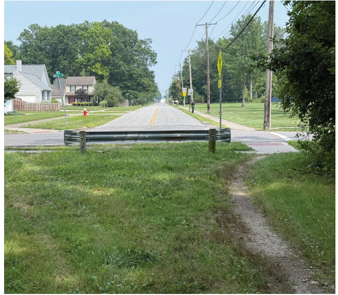
FIGURE 22 At the time of this planning process, the trail section between Forestlawn Avenue and Oster Road was not complete but still showed evidence of use. The intersection of the proposed trail with Oster Road will be a new trail head and already is used as a crosswalk.
