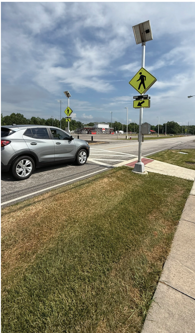
FIGURE 24 There is a rectangular rapid flashing beacon and marked crosswalk on Harris Road today between the campus and the athletic fields.
