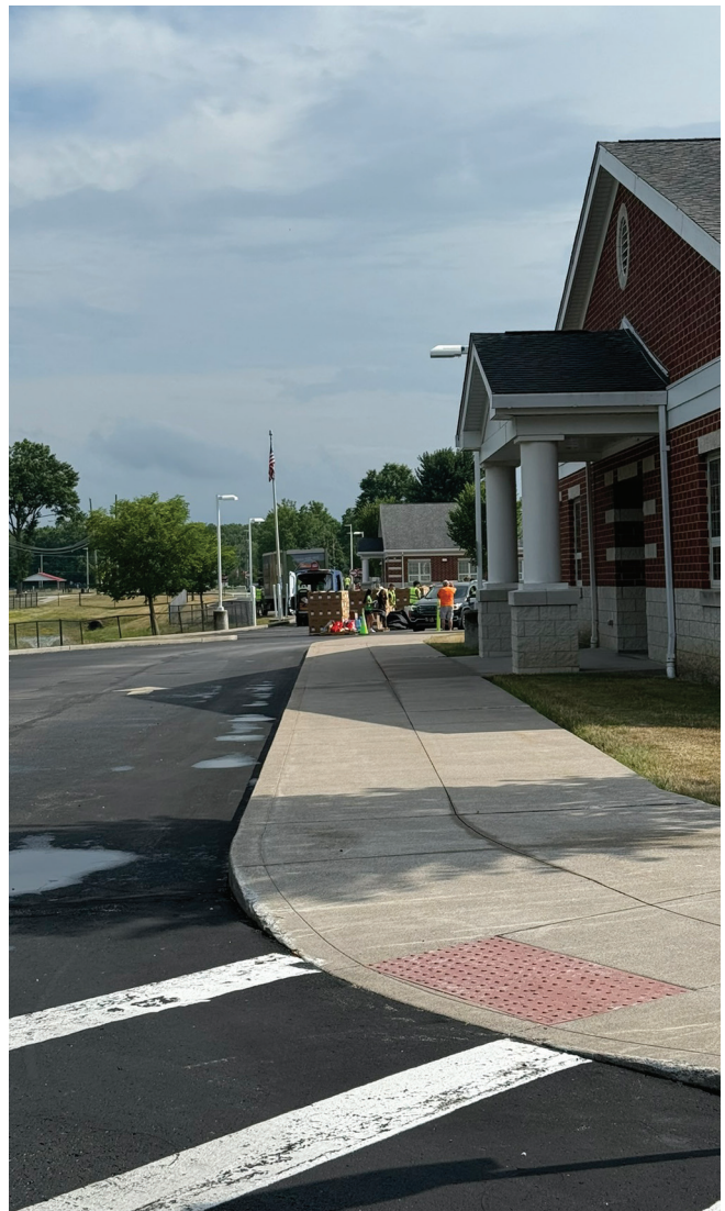
FIGURE 25 The Brookside Campus has marked crosswalks and ADA curb ramps. The campus is used for community events, like food drives, shown above.
