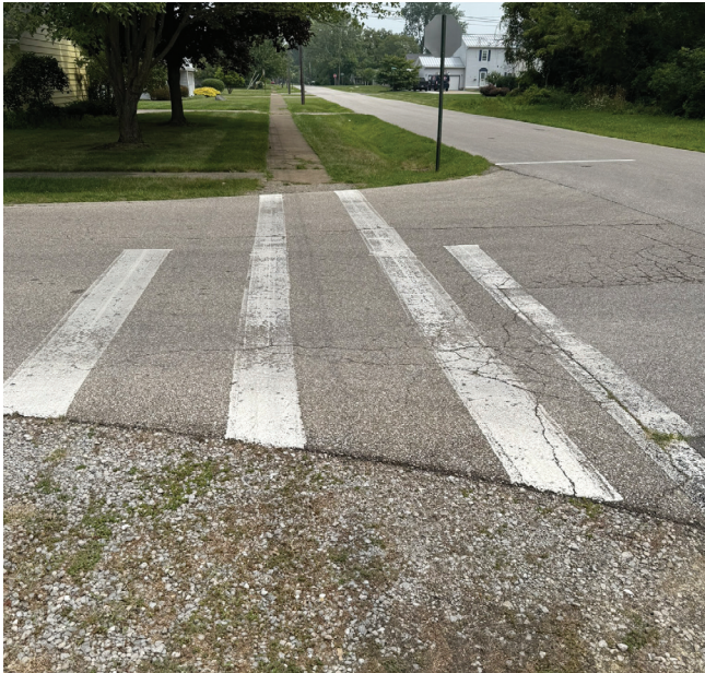
FIGURE 16 It is good that many crosswalks are marked, but the markings are not always uniform and in the correct style. This crosswalk, at the intersection of Howell Street and Ferndale Avenue has two stop bars for drivers, a narrow crosswalk, and no curb ramps. Some of these issues will be addressed over time as streets are resurfaced and brought into compliance with today's standards.
